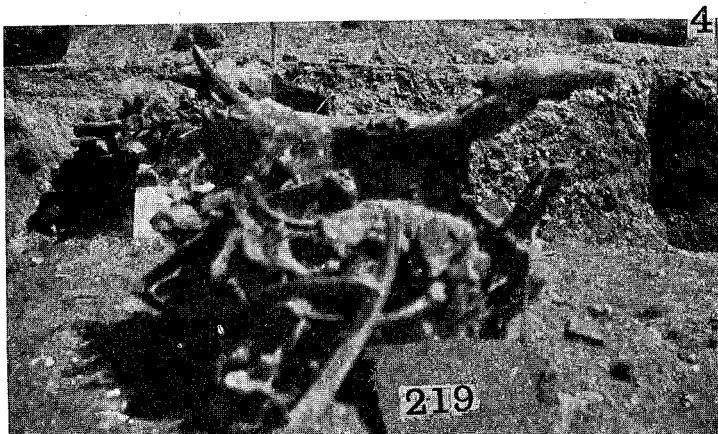
OX PILE WITH CAPPING HEAD
